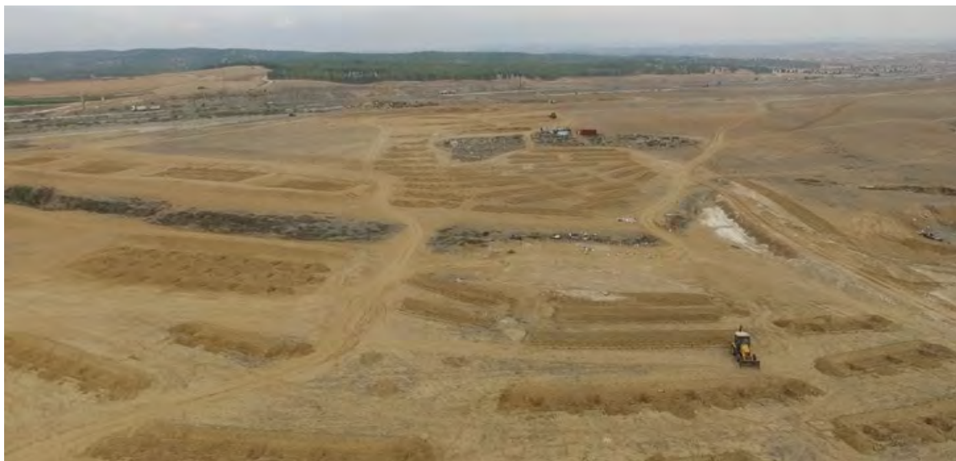
Earthworks for planting preparation in a loess area in the Northern Negev.
